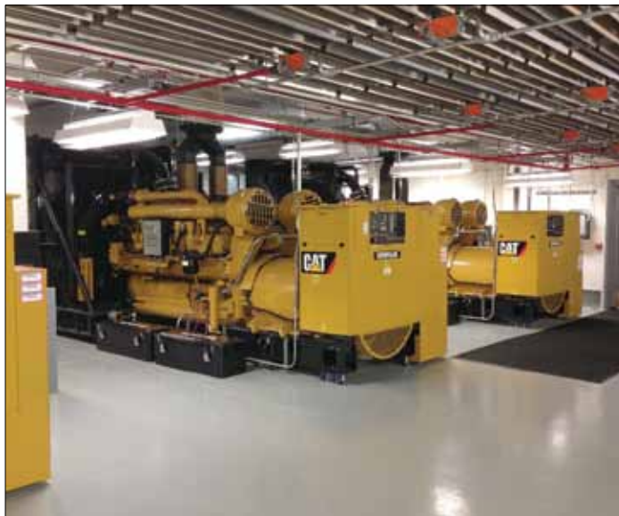
Figure 1. Generator sets housed in the data center facility. Each of the four generator sets is rated for 2 MW and is powered by a CAT 3516 engine.
