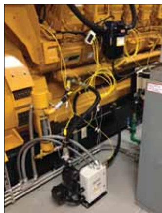
Figure 4. The test engine's right side with installed CSM and thermosiphon heater. Both heaters share a single return port using a Y-fitting.
