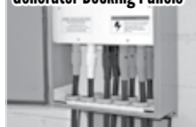
Generator Docking Panels
